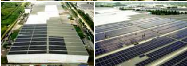
Pemasangan Solar Panel Solar Panel Installation
